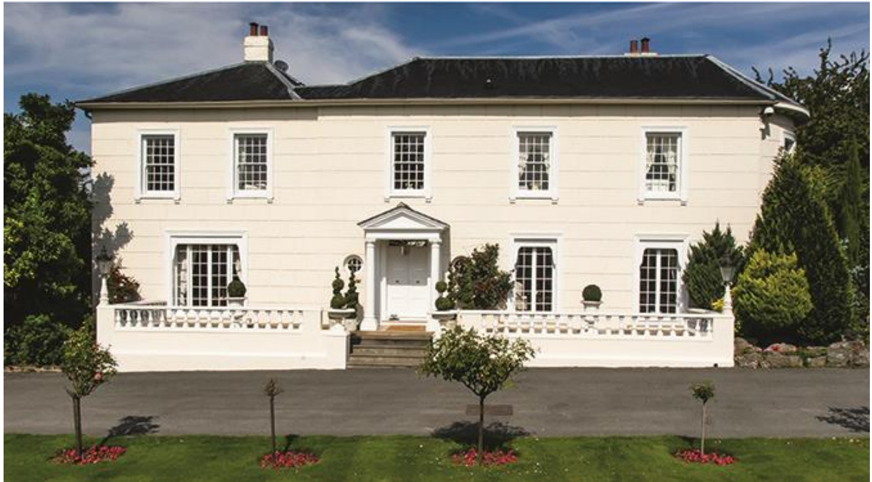
Plate 1 – The front elevation of Owls Hall.
