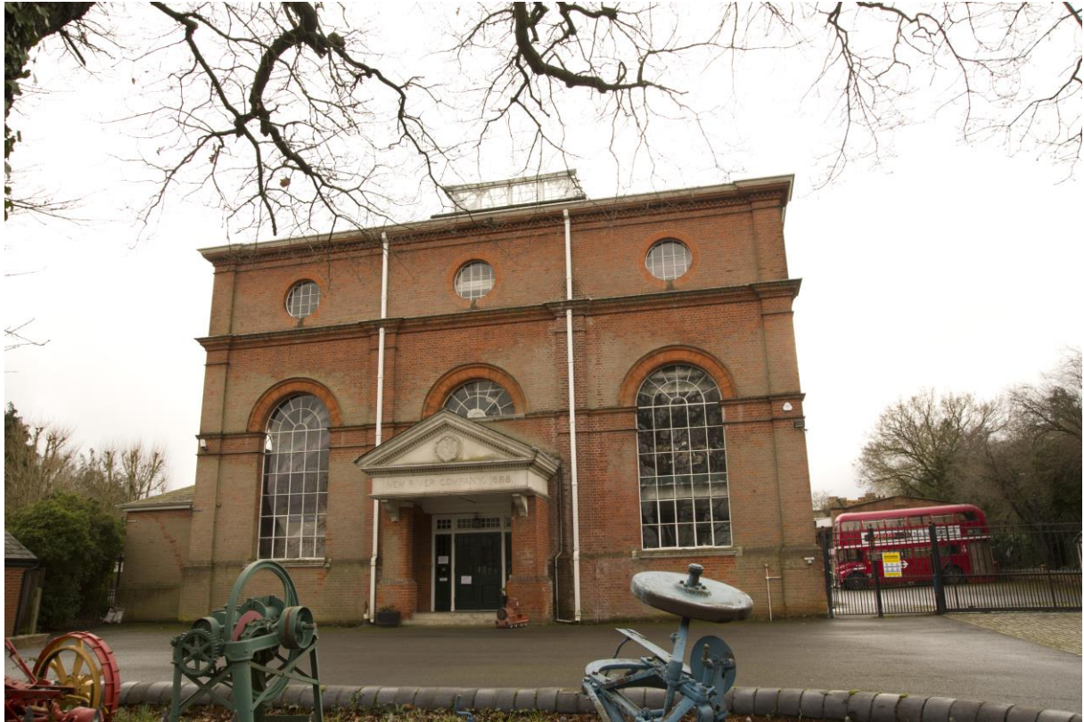
Plate 5 – Whitewebbs Road pumping station, front elevation.
