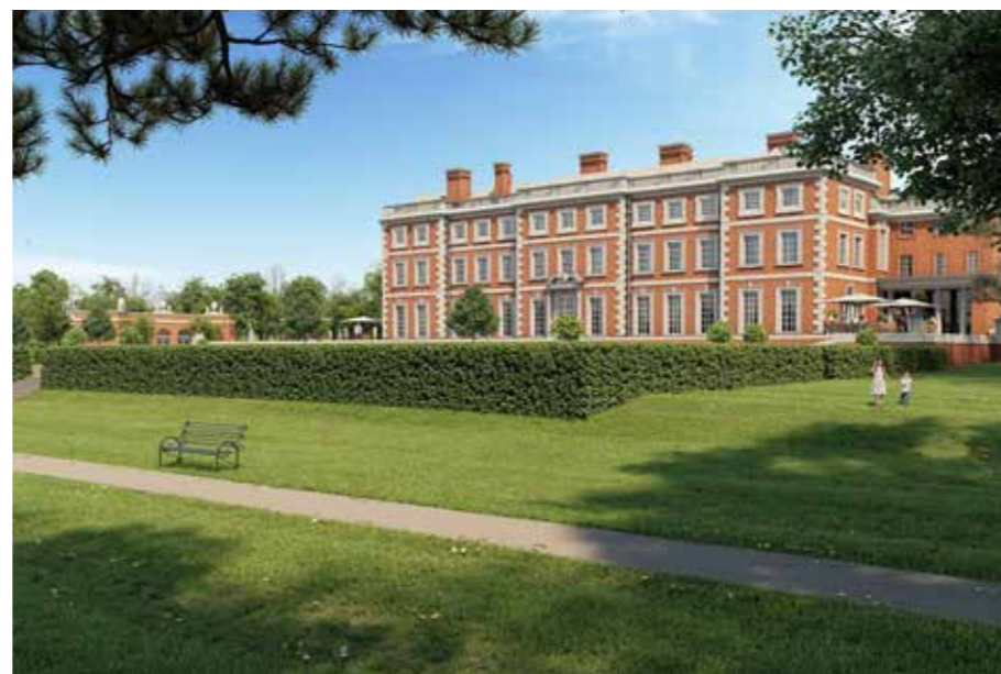
A CGI showing the redeveloped Grade II listed Trent Park House. The house is currently under development, behind scaffolding and beyond public access
