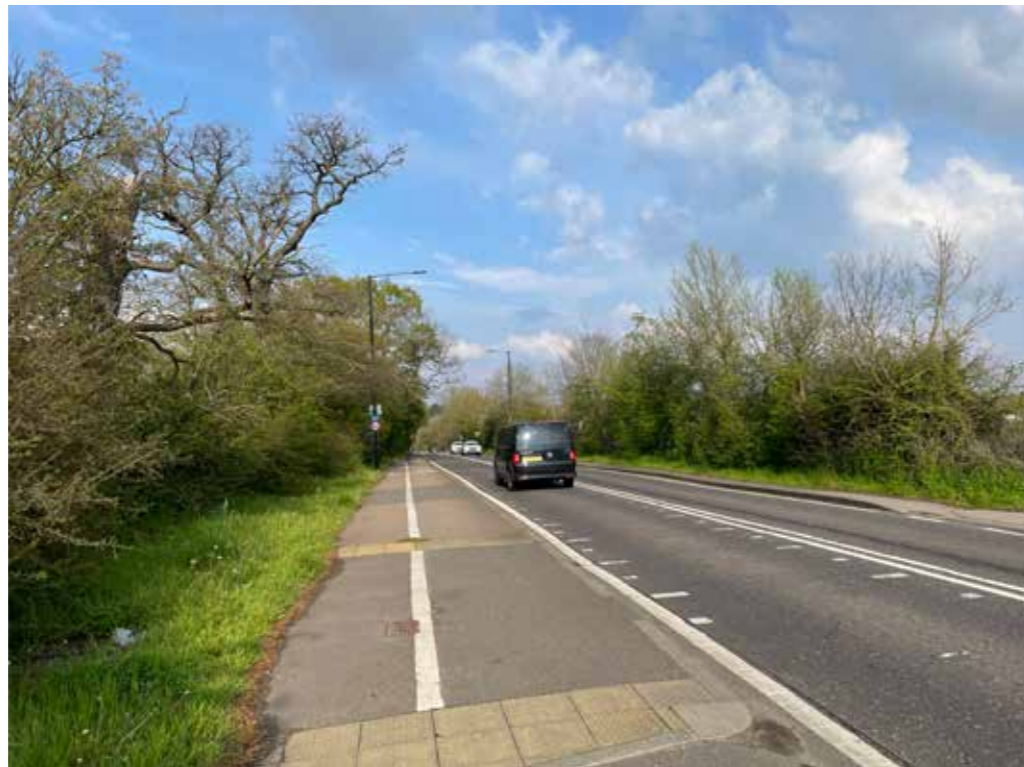
7. View looking east along A110
