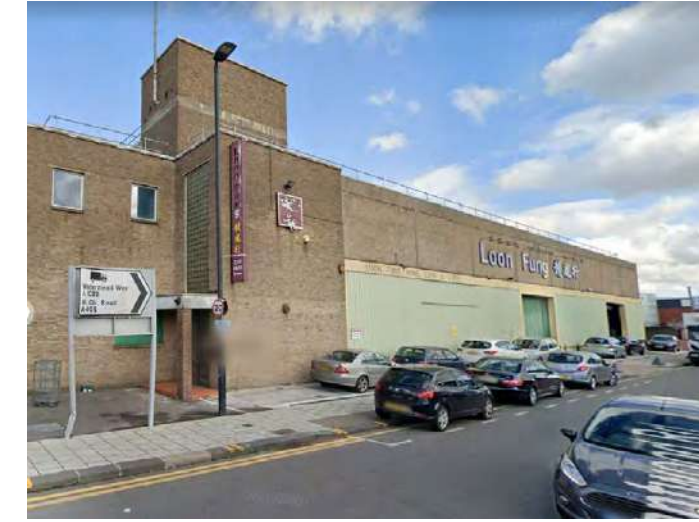
Brantwood Road Industrial Estate, Haringey
