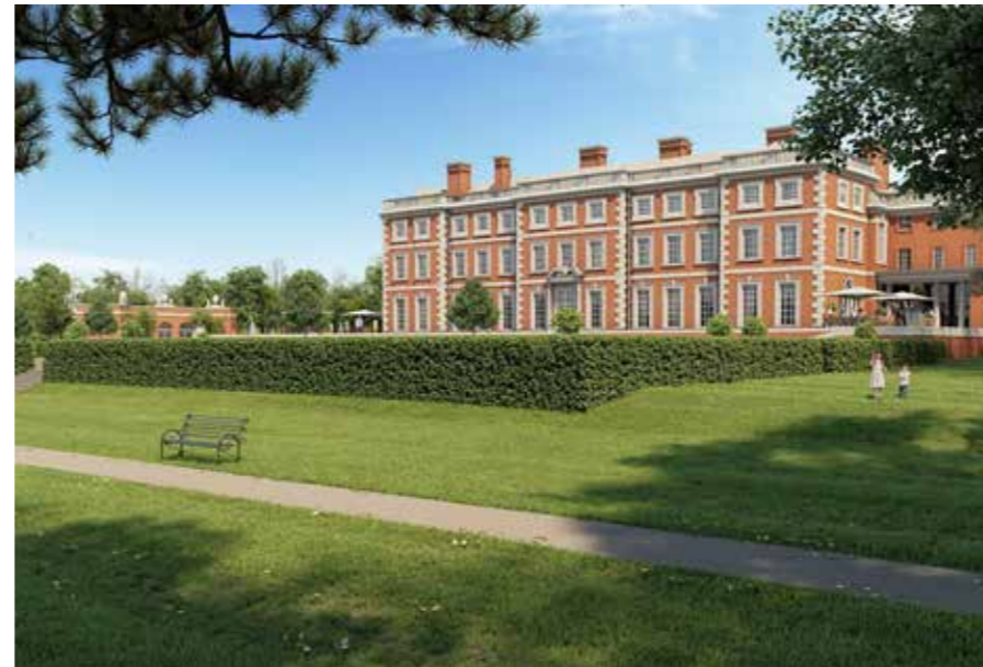
A CGI showing the redeveloped Grade II listed Trent Park House. The house is currently under development, behind scaffolding and beyond public access
