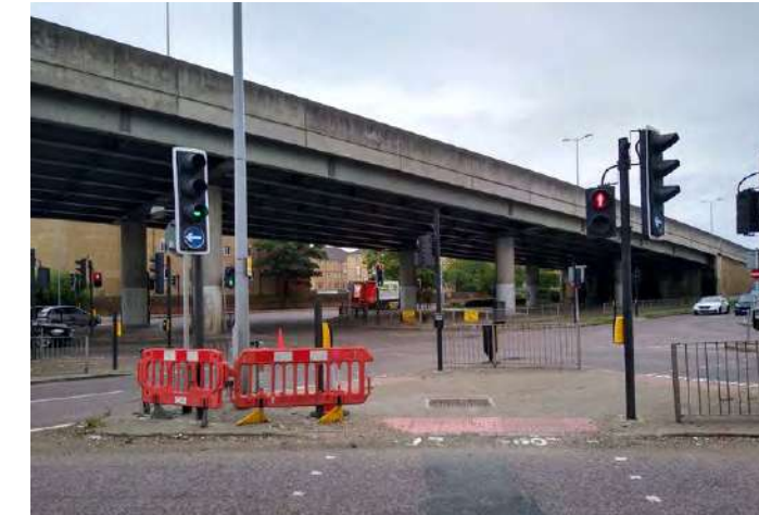
The North Circular and overpass create a significant physical barrier
