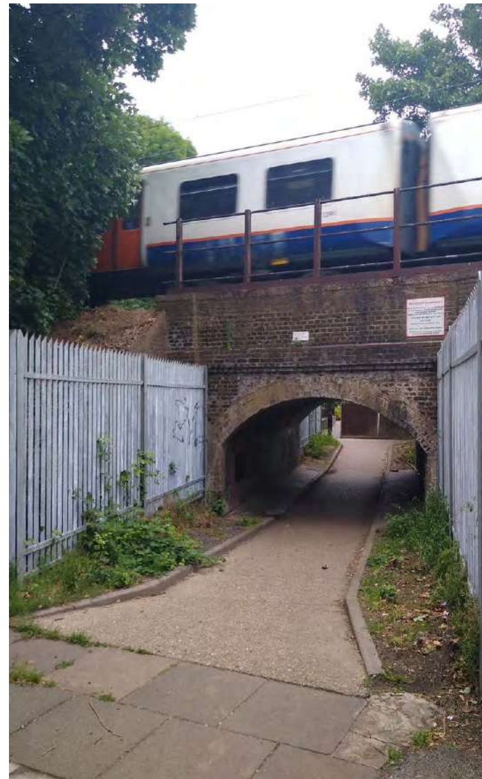
Pedestrian underpass near Warnier Drive
