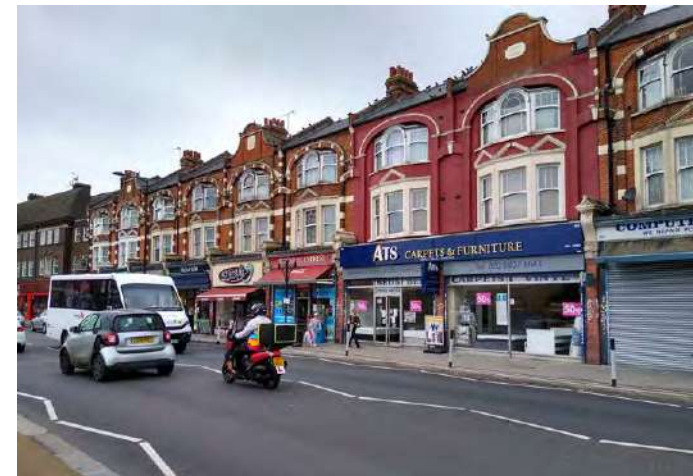
Successful independent shops along Fore Street within characterful buildings
