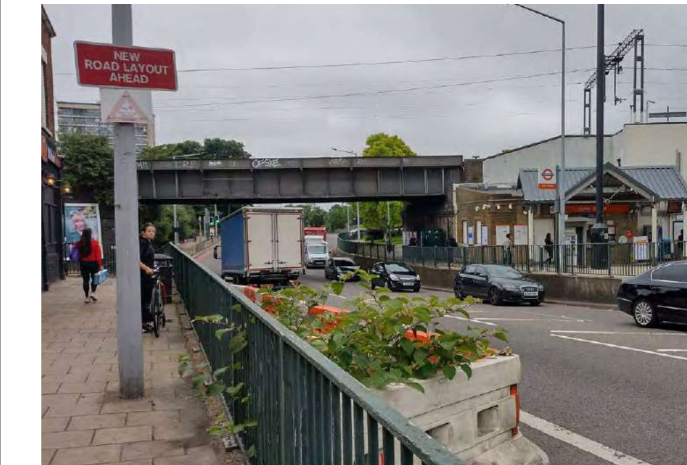
Silver Street Station - an important asset to help lever growth, stymied by the barrier created by the North Circular road
