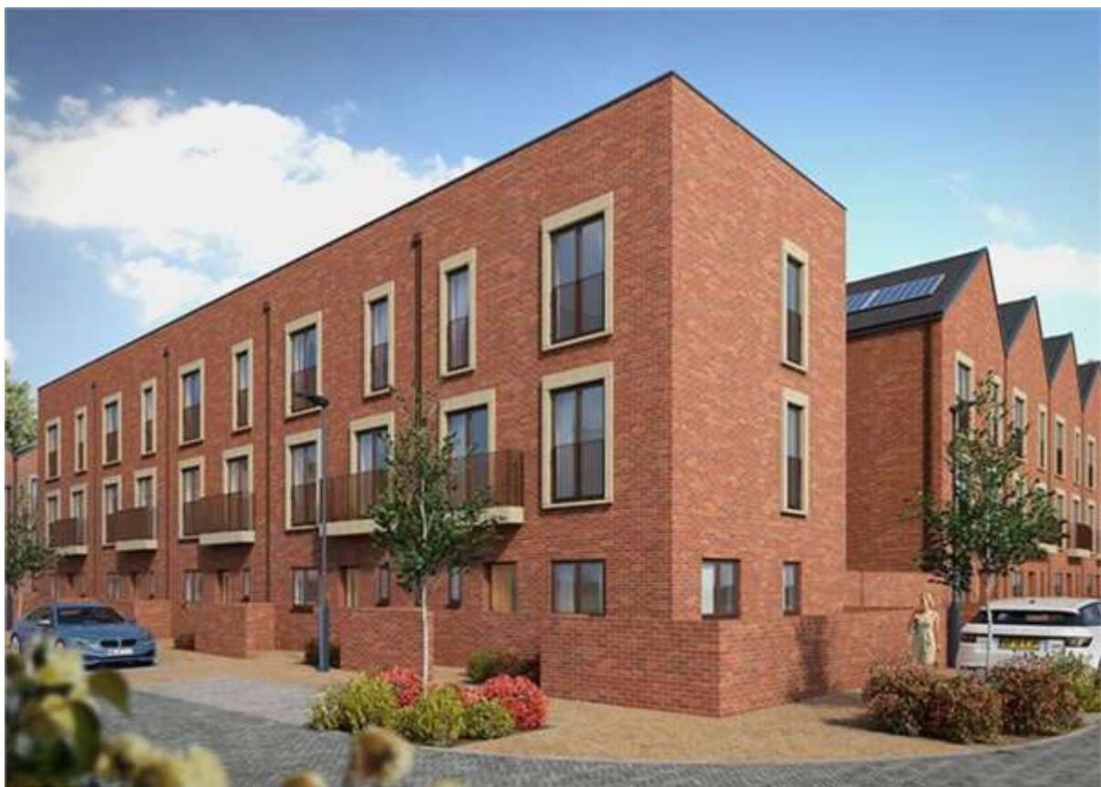
Electric Quarter Phase 1 completed in 2021
