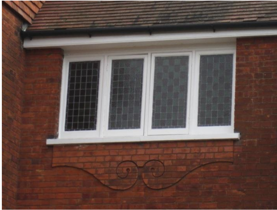
Figure 17: Crescent West, brickwork detail
