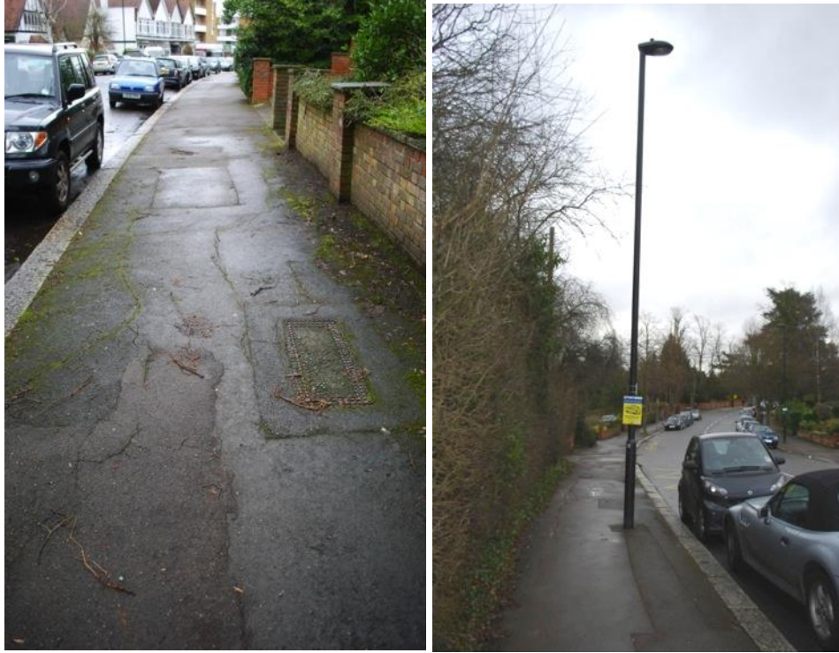
Figure 19: Footways and lamp standard
