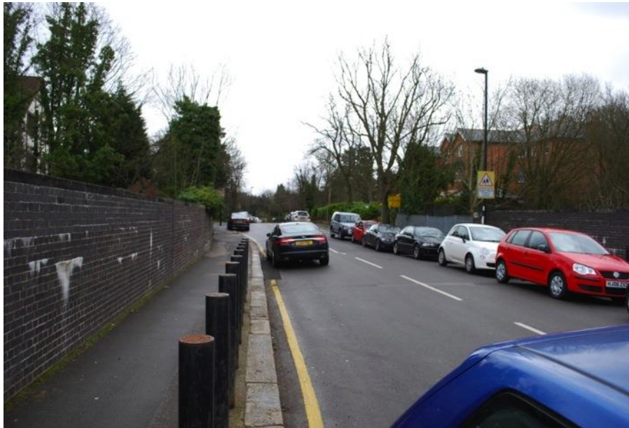
Figure 8: Bridge over railway cutting
