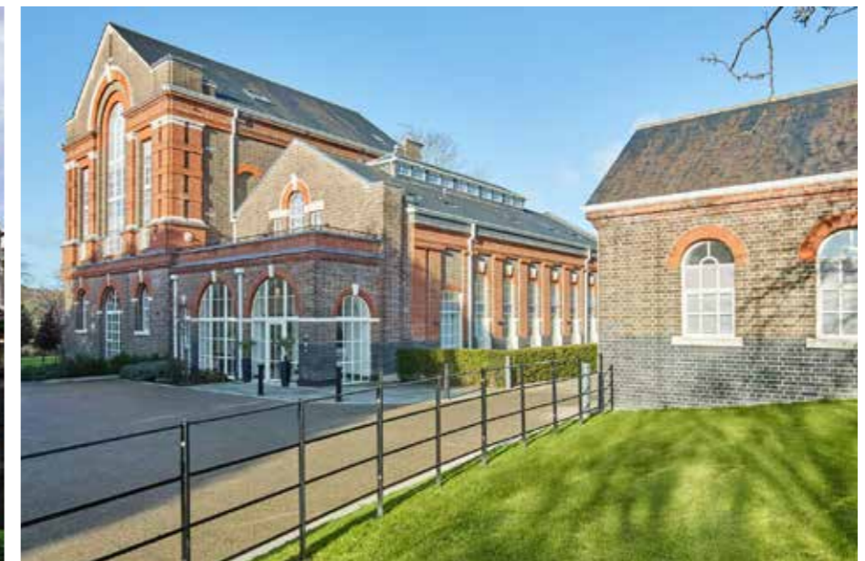
Fig. 23: Hadley Road Pumping Station
