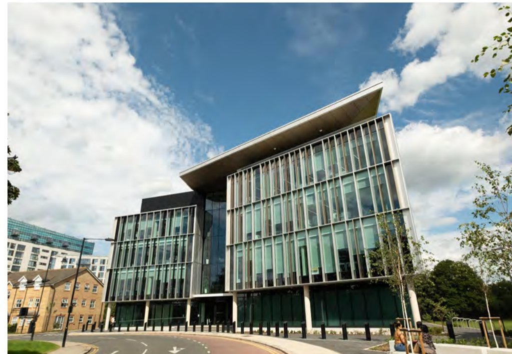
Metaswitch offices, Enfield Town
