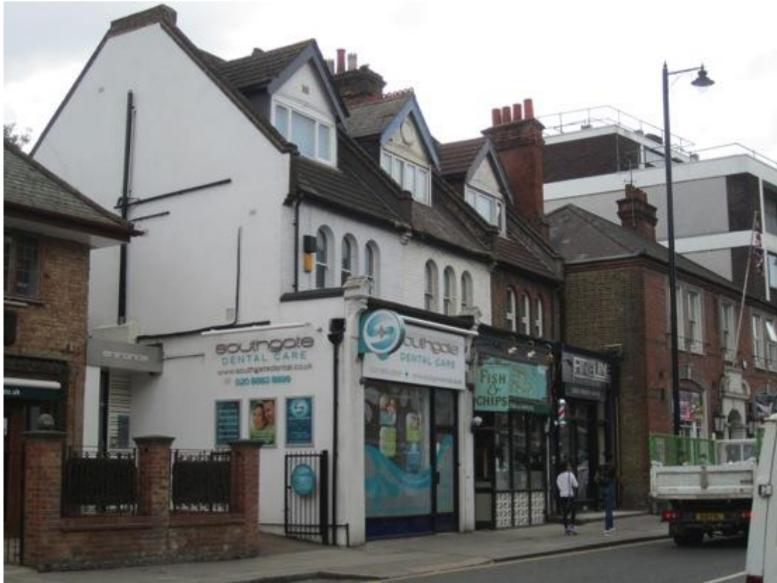
Figure 13: Shops at 11-15 Chase Side
