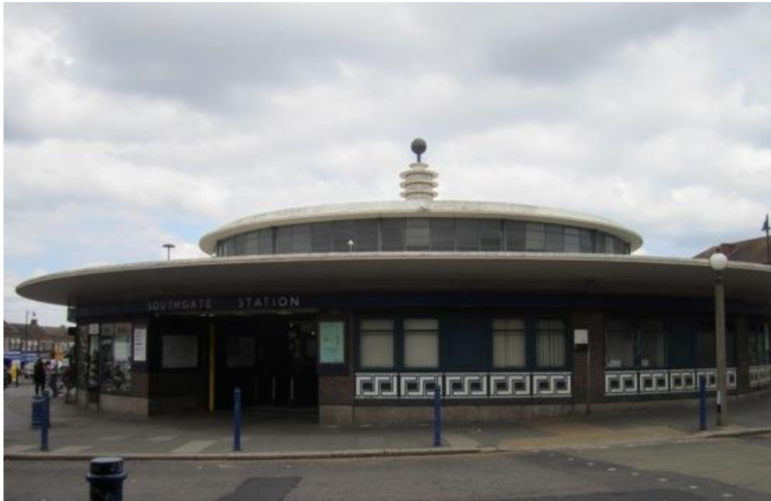
Figure 16: Southgate Station from Station Parade
