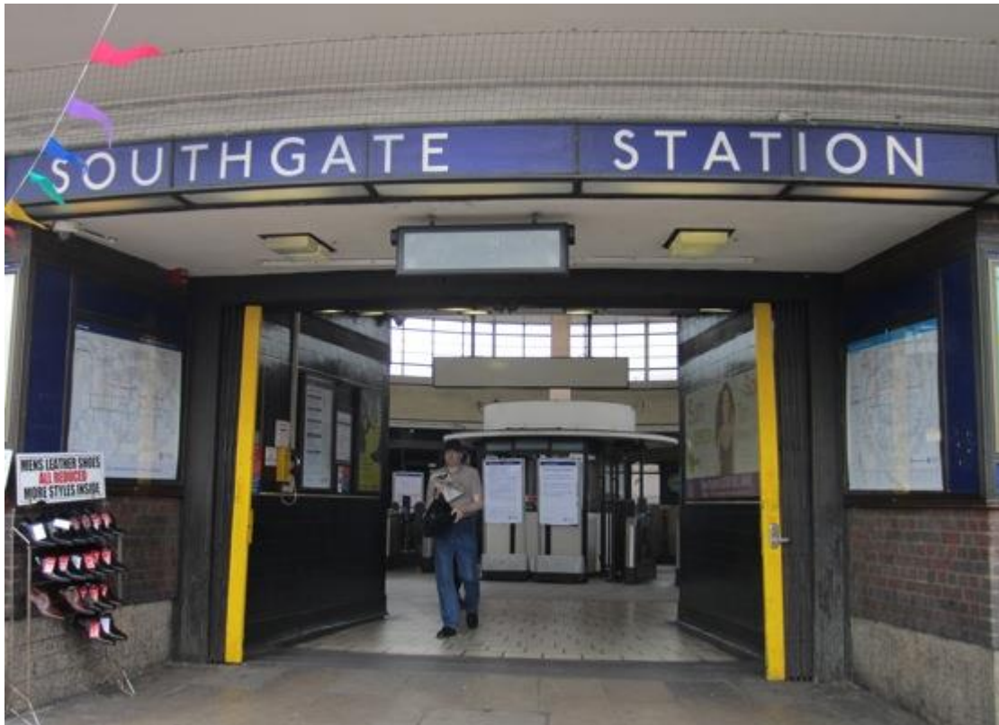
Figure 9: Southgate Underground Station, main entrance
