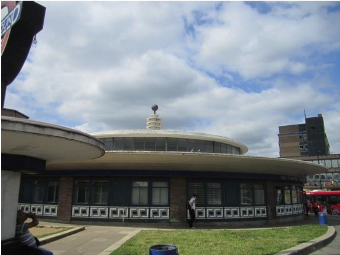
Figure 8: Southgate Underground Station from the south
