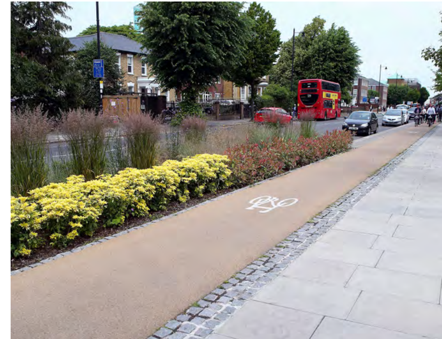
Rain Garden - London Road North
