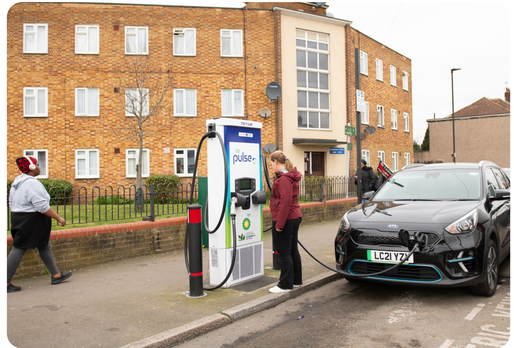
Electric vehicle charging point
