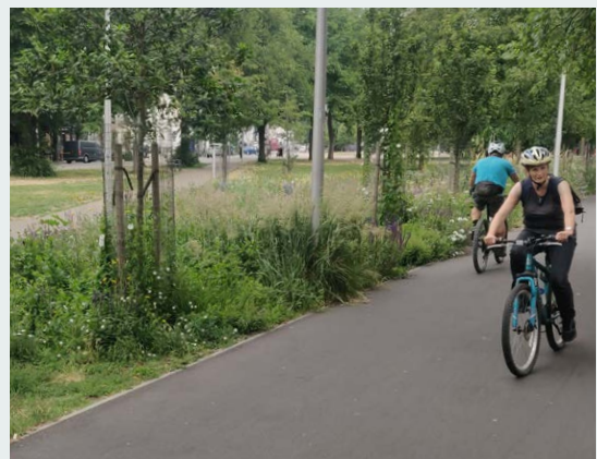
Segregated cycle lane as part of wider traffic and public realm improvements - Valley Gardens, Brighton
