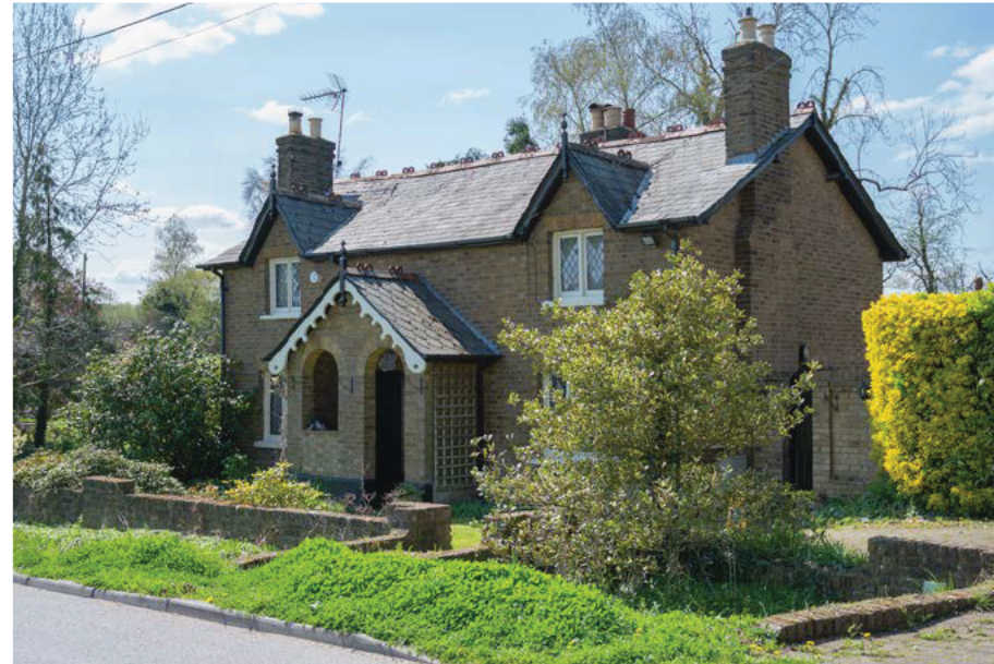
Fig. 27: Looking southwest on Burntfarm Ride Lane, showing former workers cottages associated with Theobalds Farm. Located within the proposed Crews Hill site boundary
