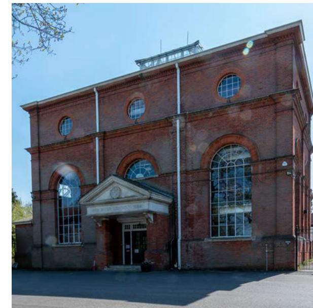
Fig. 22: Former New River Pumping Station (1898)
