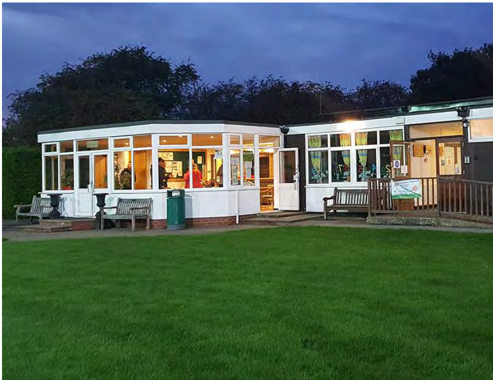
Figure 39: Hadley Wood Association Centre (source: Troy Planning)
