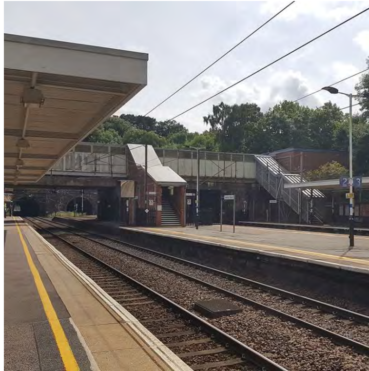
Figure 41: Hadley Wood railway station (source: Troy Planning)
