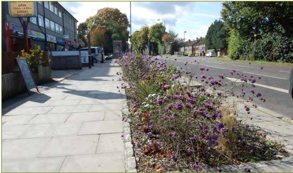
Figure 30: Rainwater gardens in Oakwood, Enfield, part of the SuDS network (source: Enfield Council)
