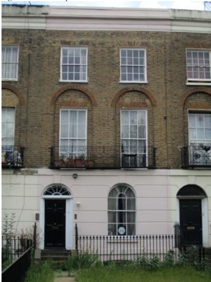
Figure 15: No. 98, with small pane glazing
