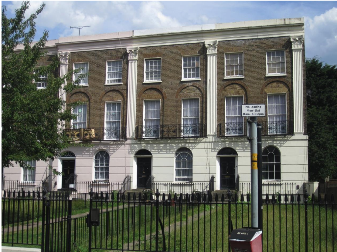
Figure 14: Southern pavilion block
