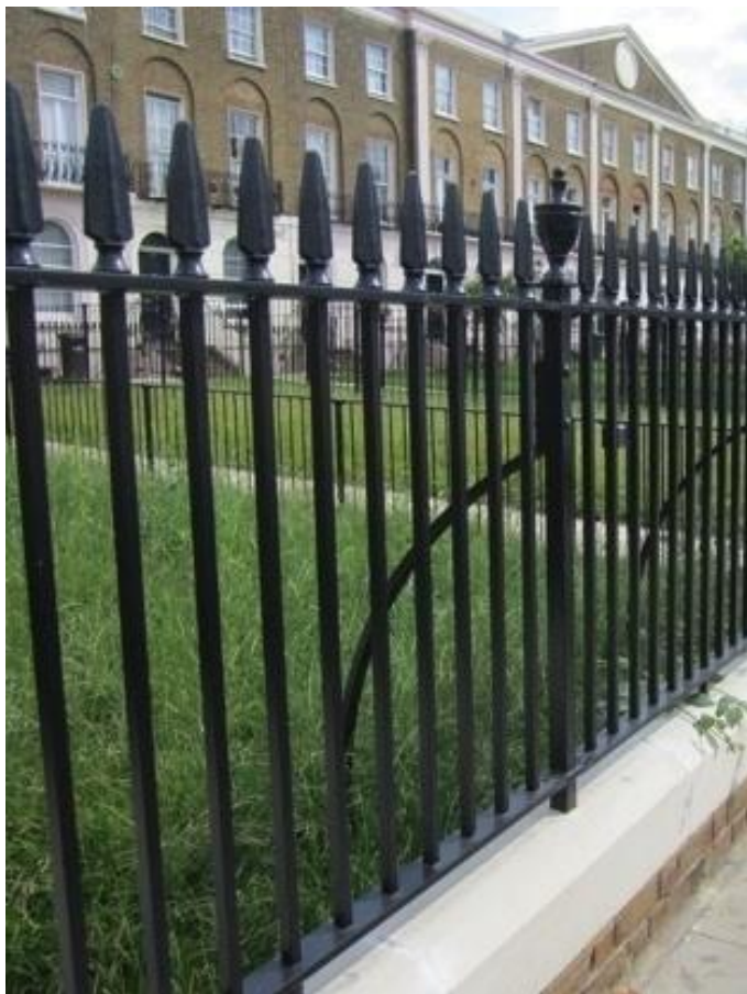
Figure 17: Railings and plinth wall, 2013-14
