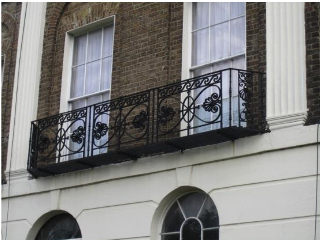
Figure 11: Early 19th century wrought iron balcony, No. 84
