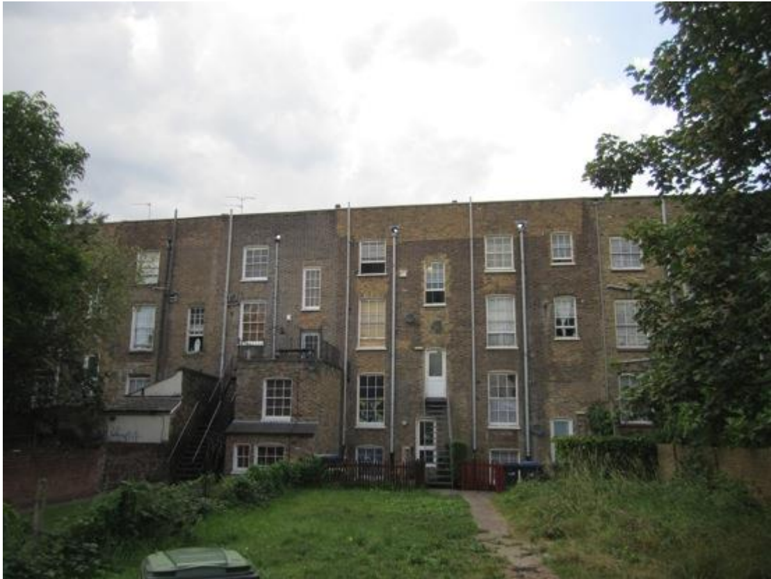
Figure 19: Rear elevation showing later extensions and altered fenestration
