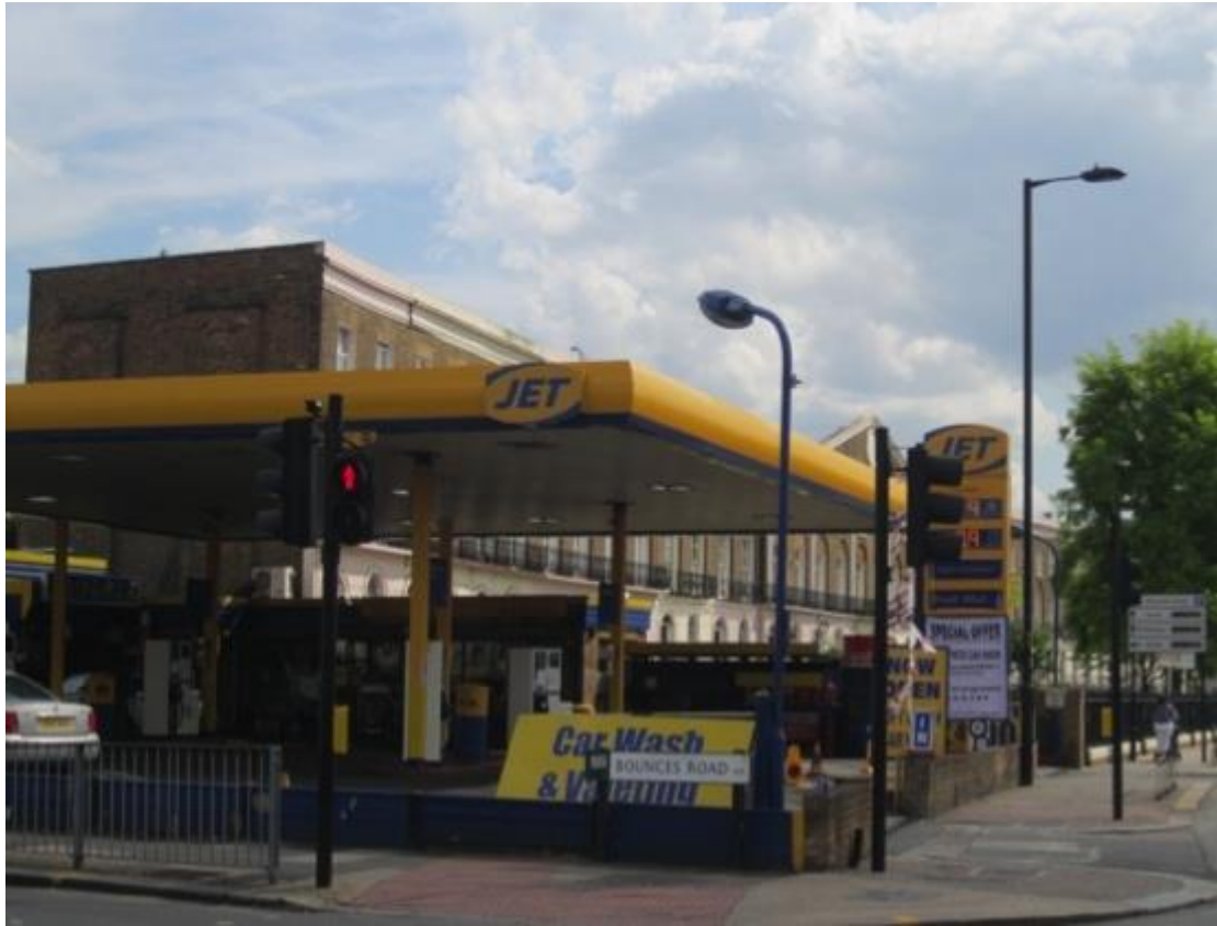
Figure 16: Petrol filling station, corner Bounces Road and Hertford Road
