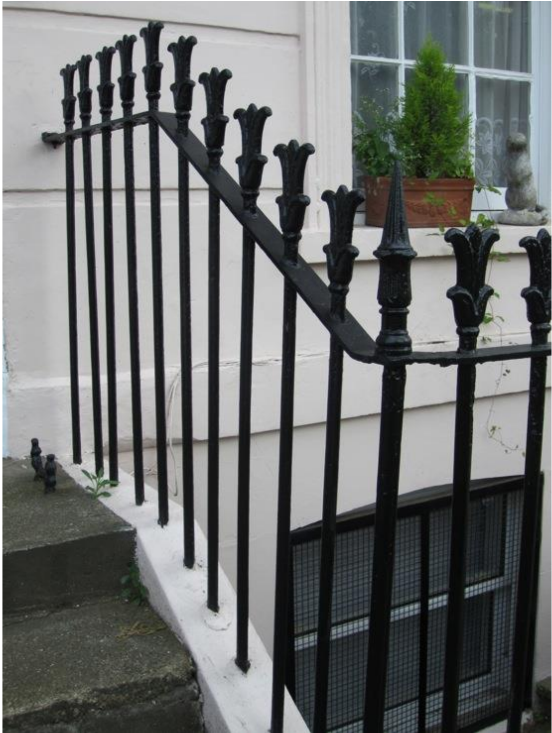
Figure 22: 19th century railings and boot-scraper
