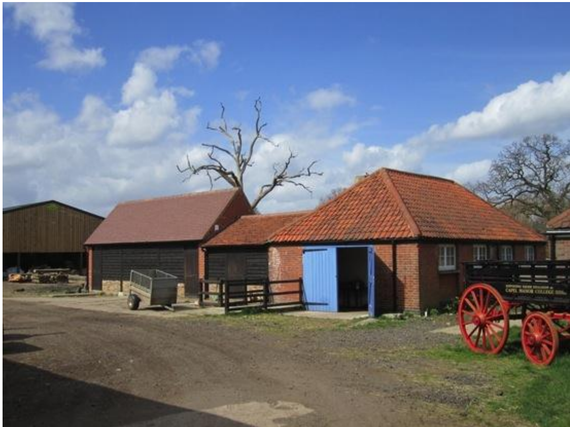
Figure 15: Repaired farm buildings
