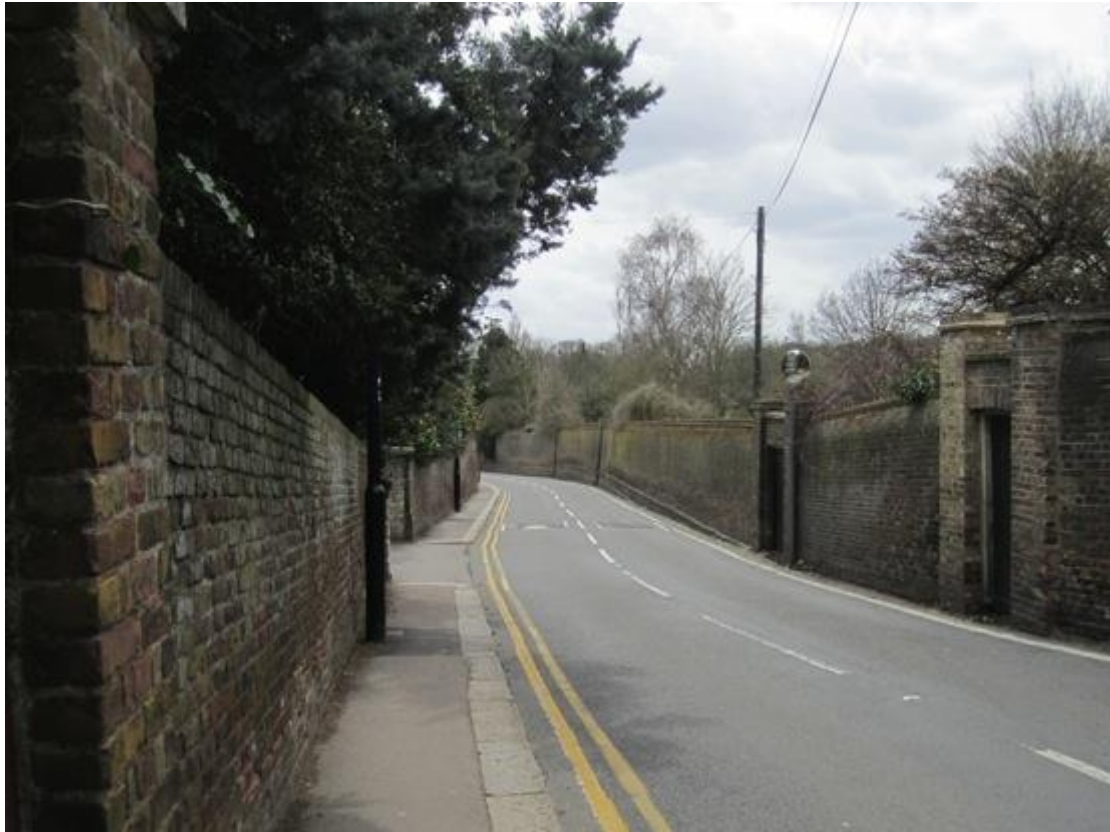
Figure 41: Boundary Wall to Myddelton House (to right)
