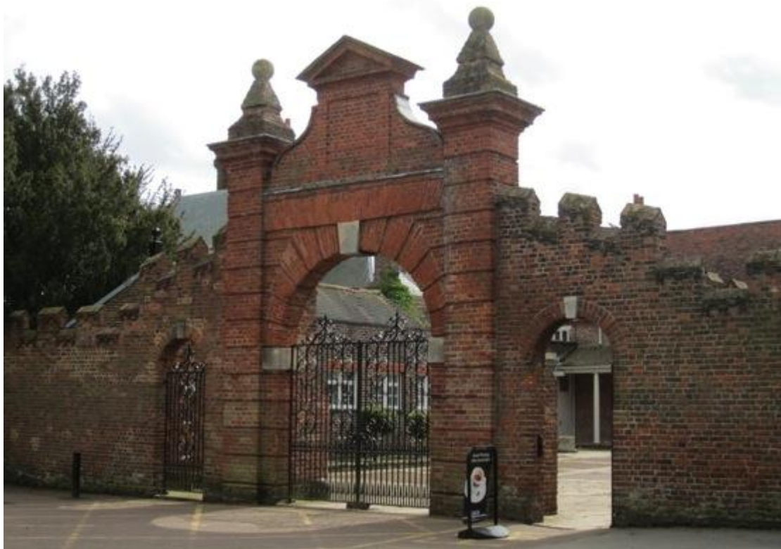
Figure 14: Entrance to the service court
