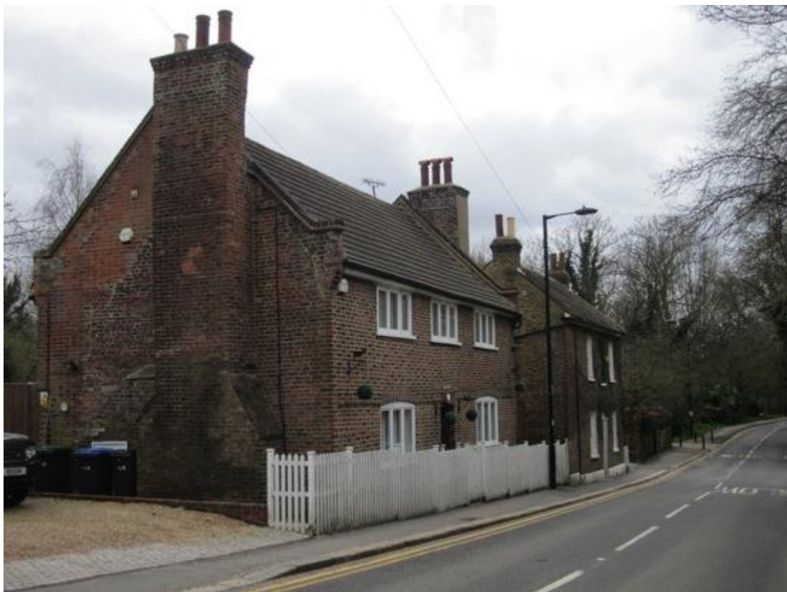
Figure : 5 and 6 Maiden's Bridge Cottages
