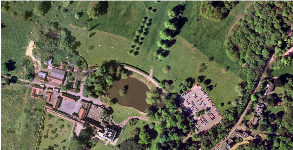
Figure 20: Aerial photograph showing impact of car park
