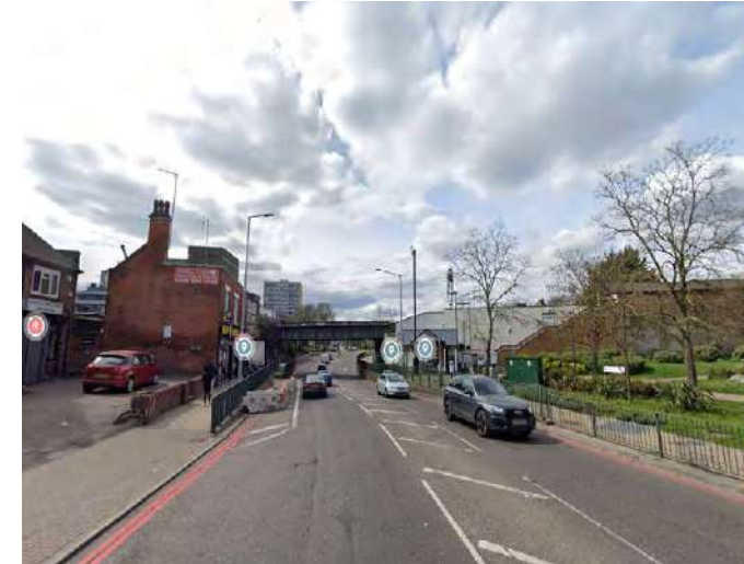
Existing condition at Sterling Way
