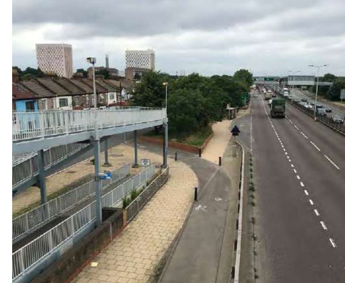
Existing pedestrian crossing in Kenninghall underpass looking North
