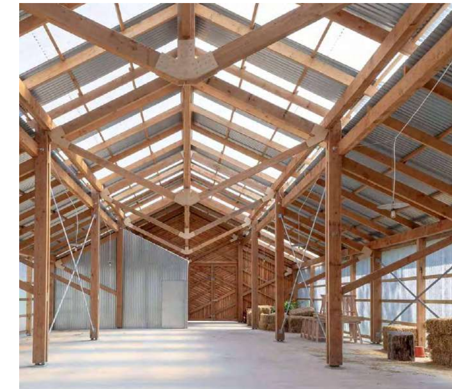
Waterloo city farm, community farm and studio located on previously waste land site - Feilden Fowles
