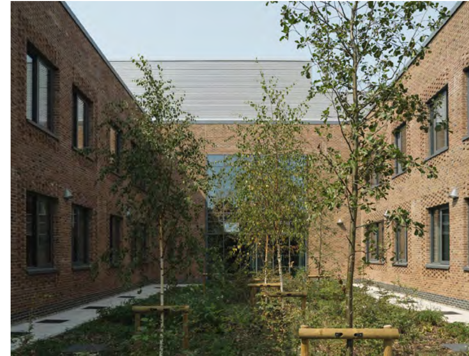
Inpatient facilities at St Anns hospital Haringey, people focused health care facilities including Adult Acute ward, Eating Disorders ward, with shared accommodation including visiting space, staff rest room and a multi-faith room - Medical Architecture
