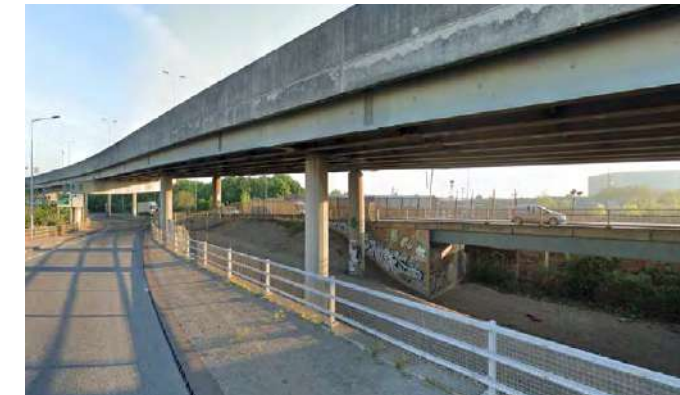
Existing NC Flyover and underpass condition
