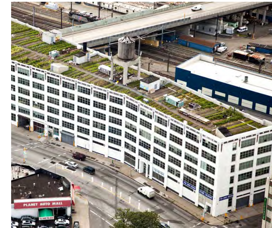
Green Rooftops - Brooklyn Grange productive rooftops
