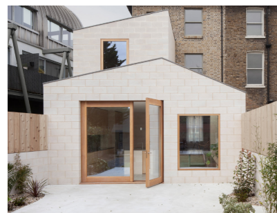
Rear extension, Camden
