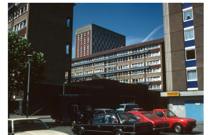
The site in 1988, with a podium between Hereford Hse. and Leicester Hse.
