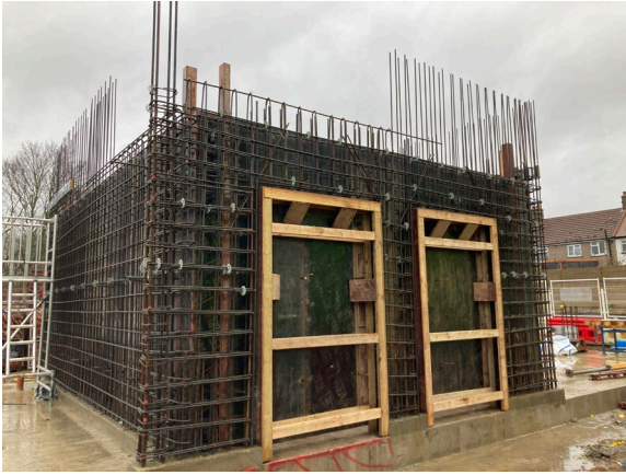
Picture 2: Ground floor walls and columns
