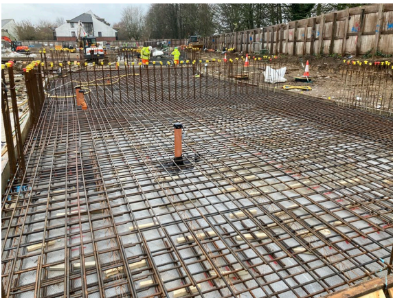
Picture 3: Ground floor slab steelwork
