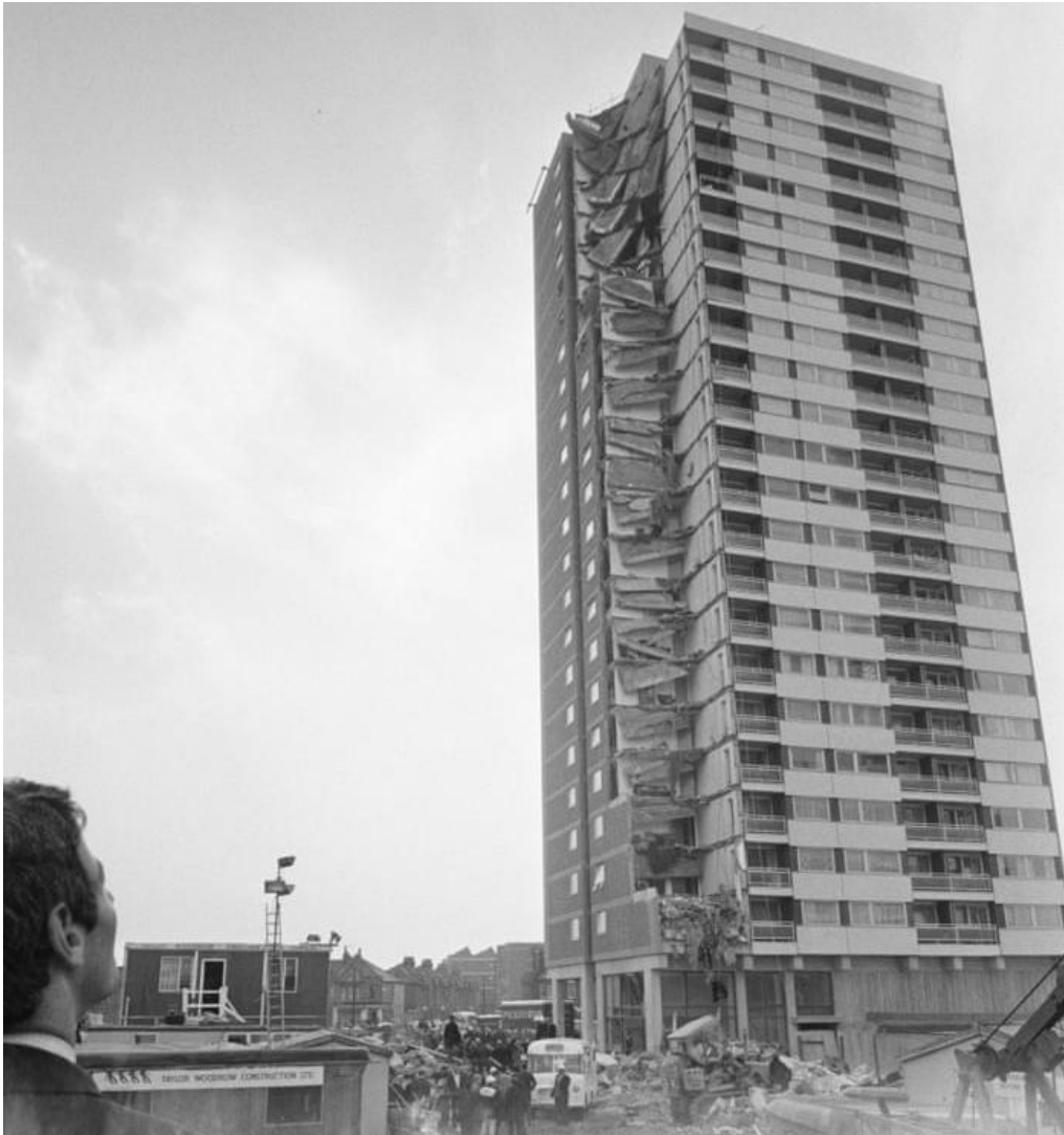
Figure 5 – The collapse of Ronan Point in 1968 (The Guardian, 2018)
