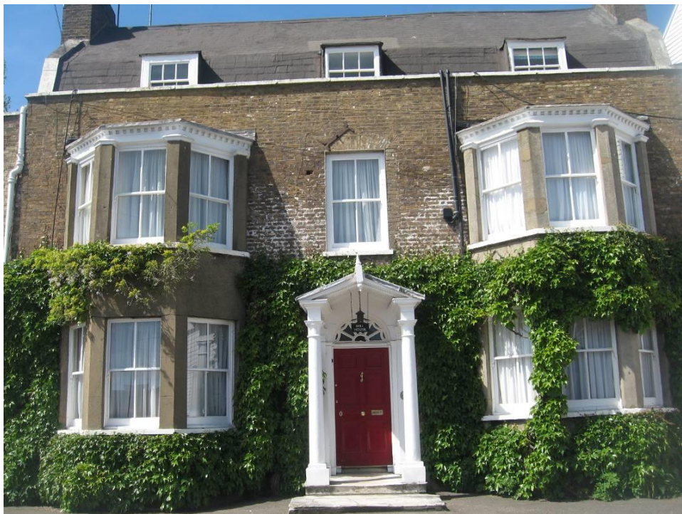
Figure 8: Mill House, south elevation
