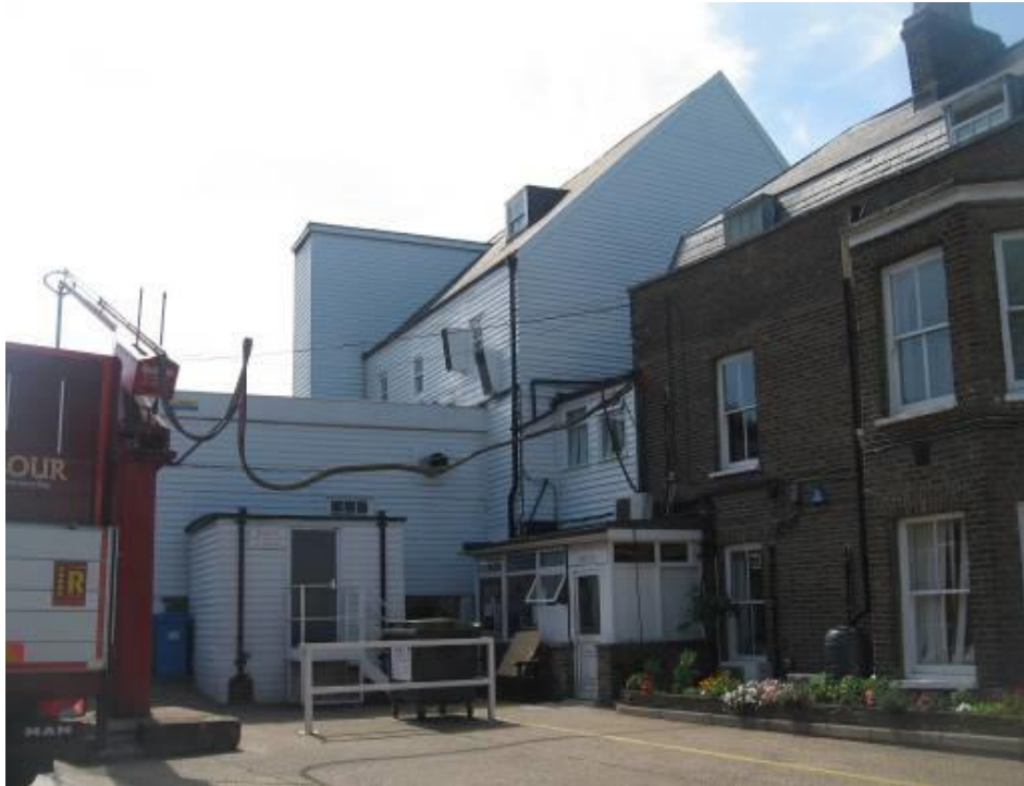
Figure 18: Additions to mill frontage
