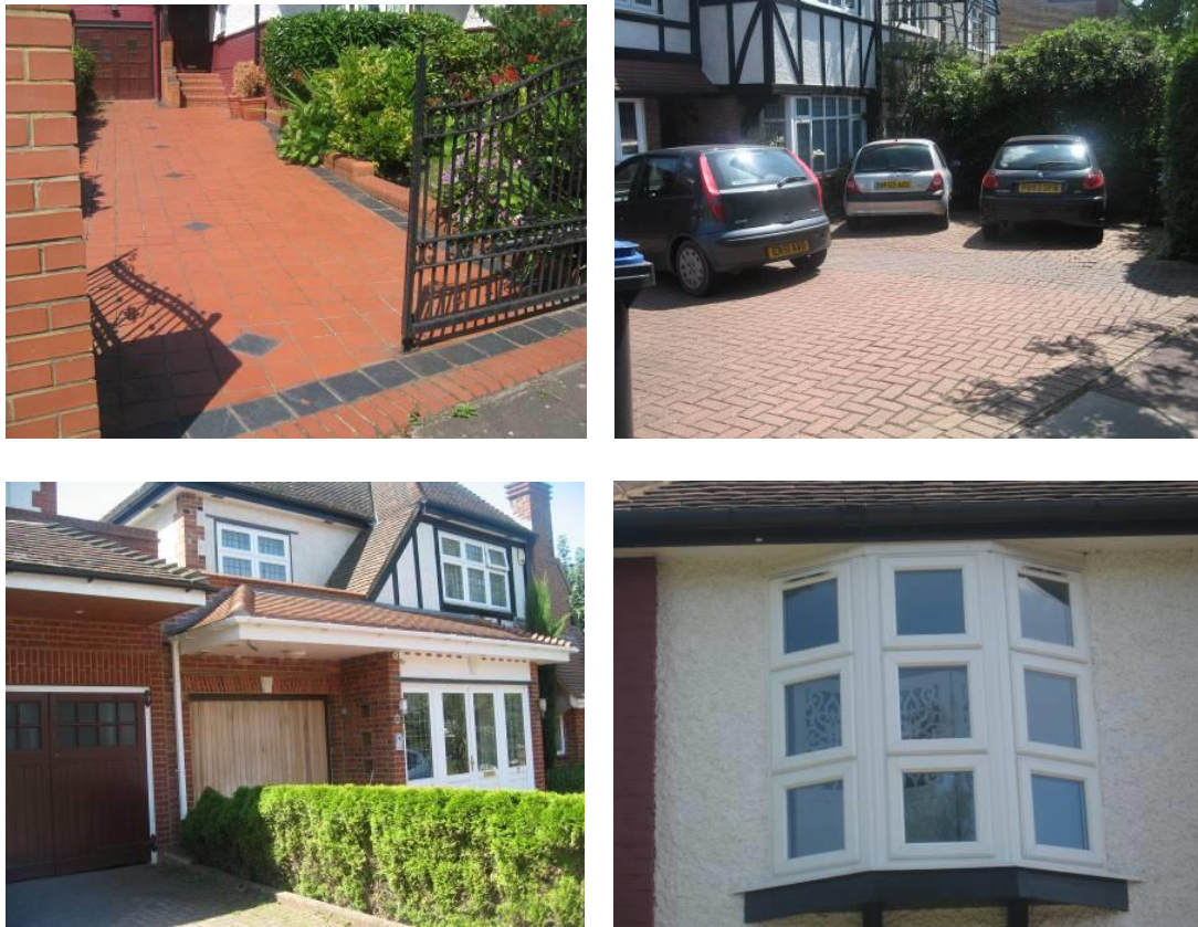
Figure 10: Unsympathetic changes to settings and replacement of original features
