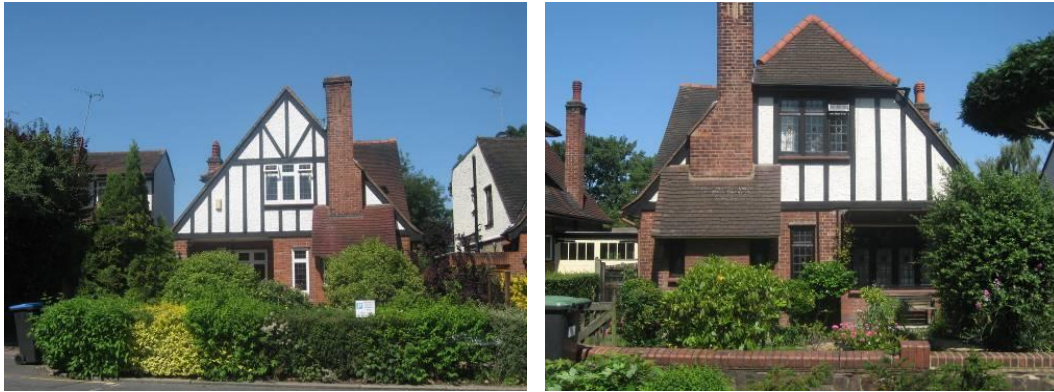
Figure 6: Two styles of the 'cottage house' with front chimney stack - gabled (left) and half-hipped
