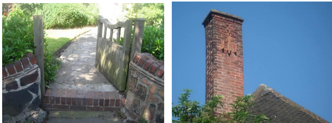
Figure 8: Original boundary walls and traditional oak gate; and (right) tile detail to a tall stack
