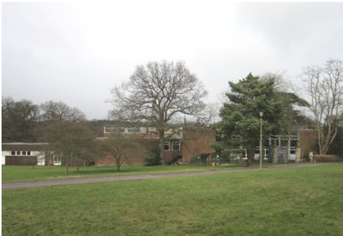
Figure 19: Jebb Block looking south
