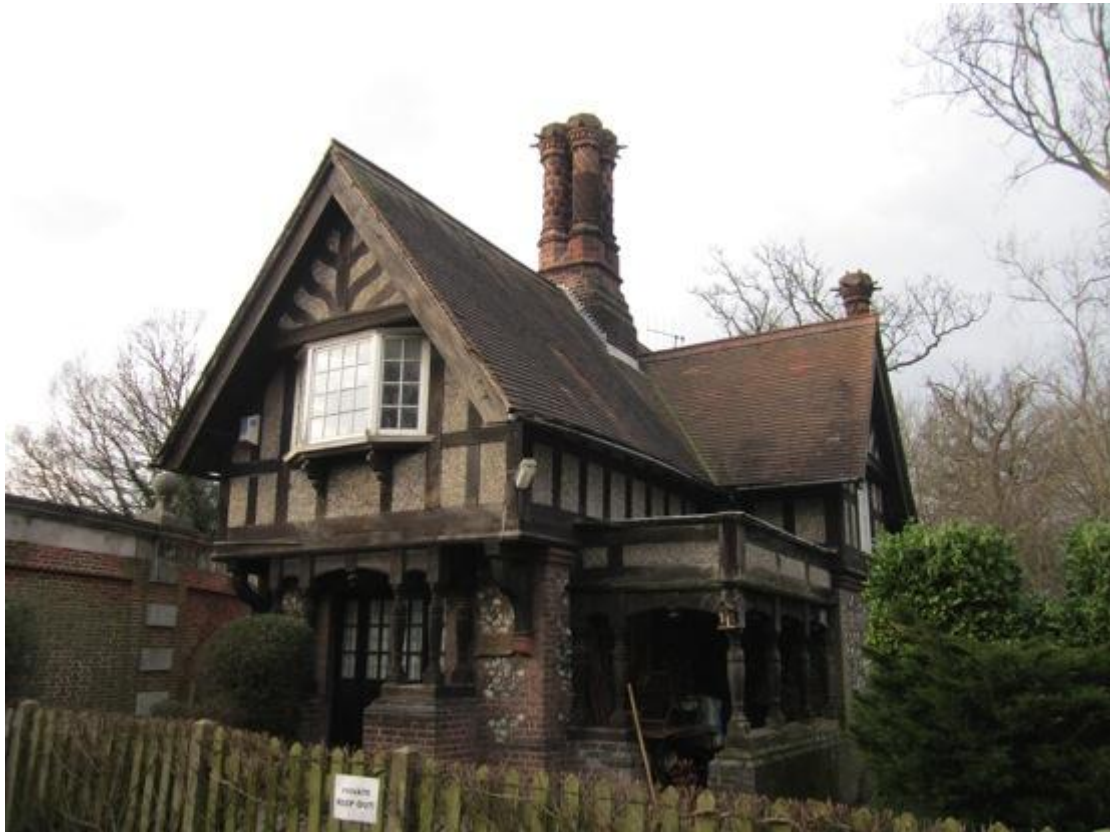
Figure 30: West (Front) Lodge
