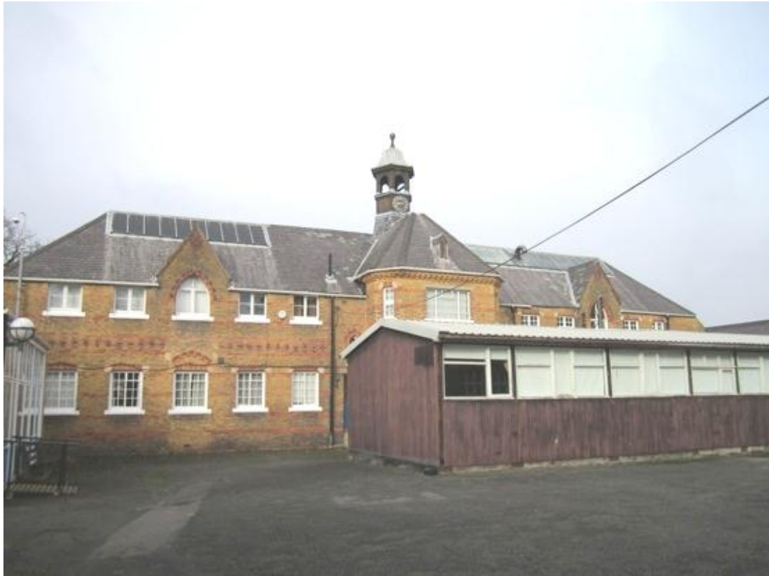
Figure 14: Stable court yard
