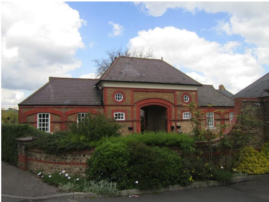
Figure 15: Former Ambulance Station
