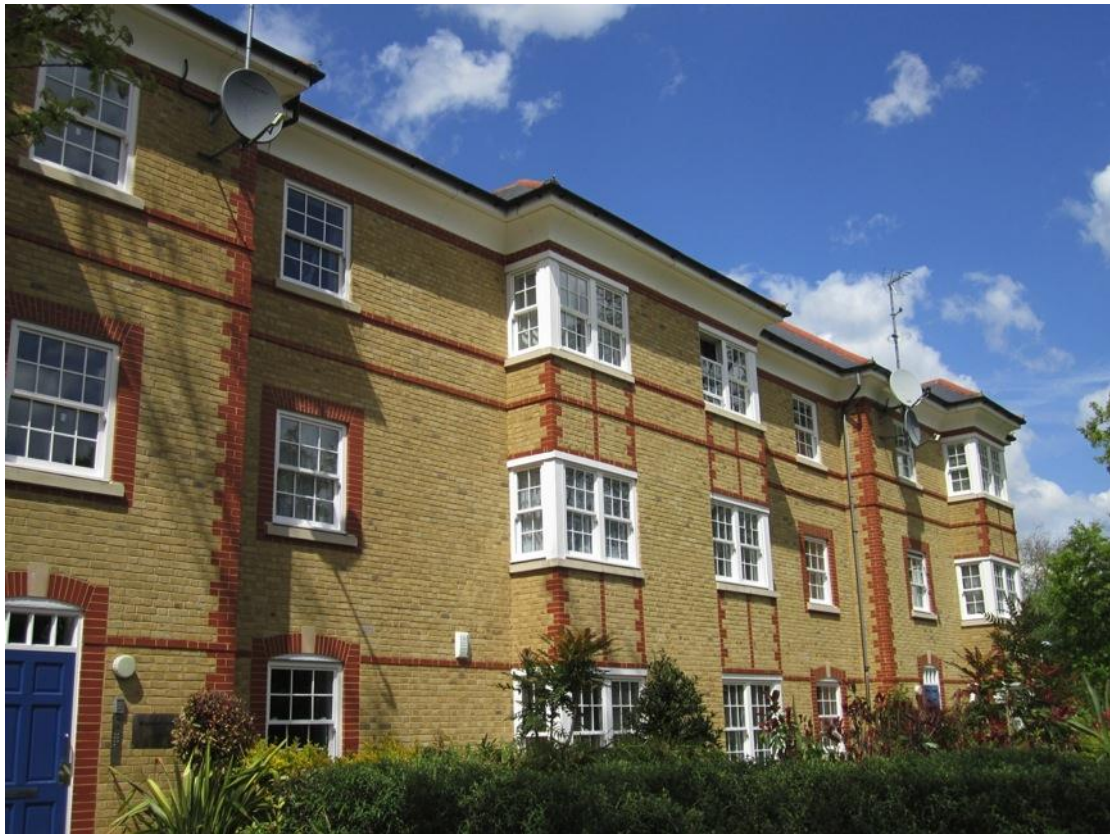
Figure 17: Flats on the site of the 1970s Health Centre
