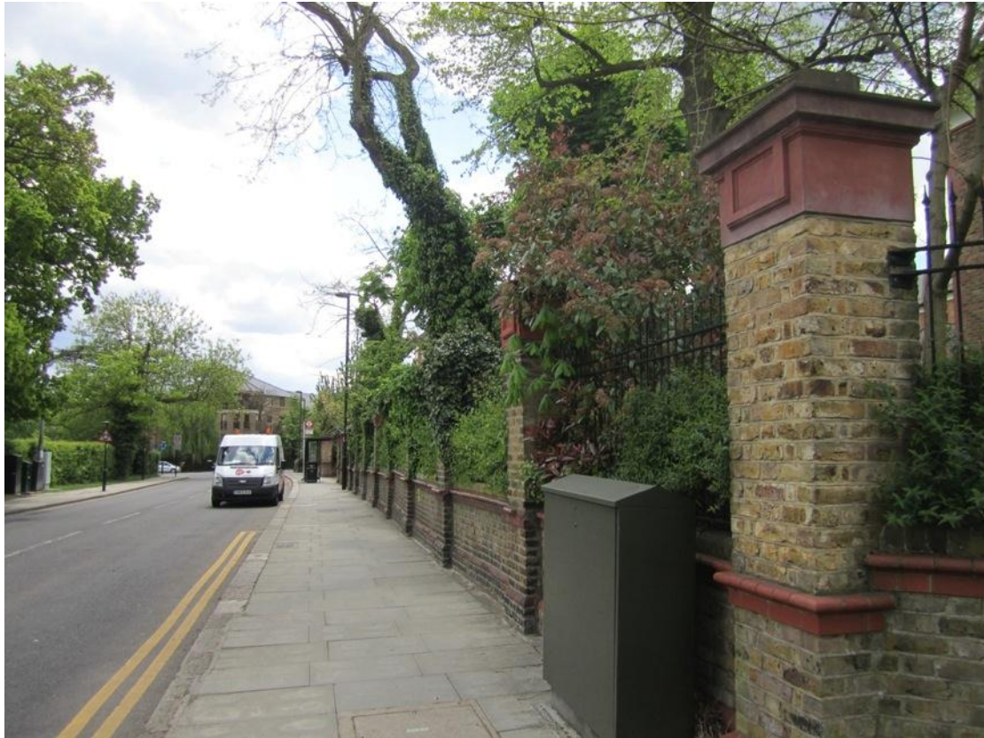
Figure 14: Worlds End Lane, boundary wall
