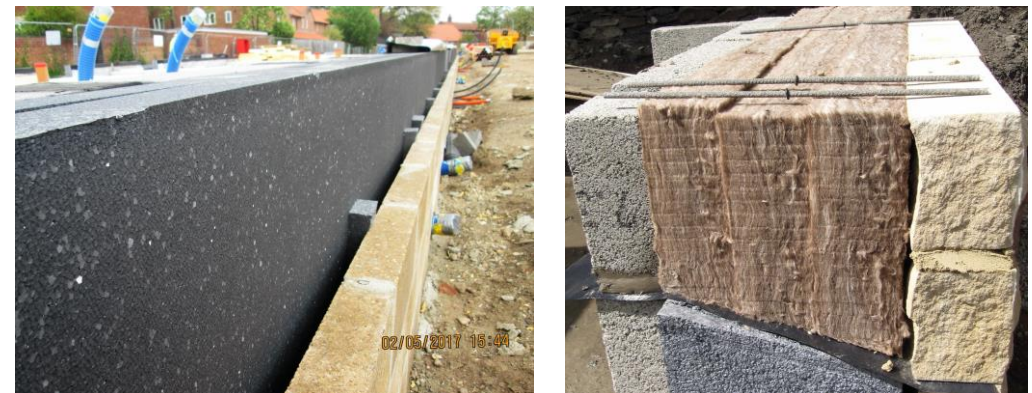
Figure 11.15 - Good examples of insulation installed on site, showing methods to eliminate gaps (wedging and overfilling). Left: Goldsmith street © Etude, Right: © Green building store.
