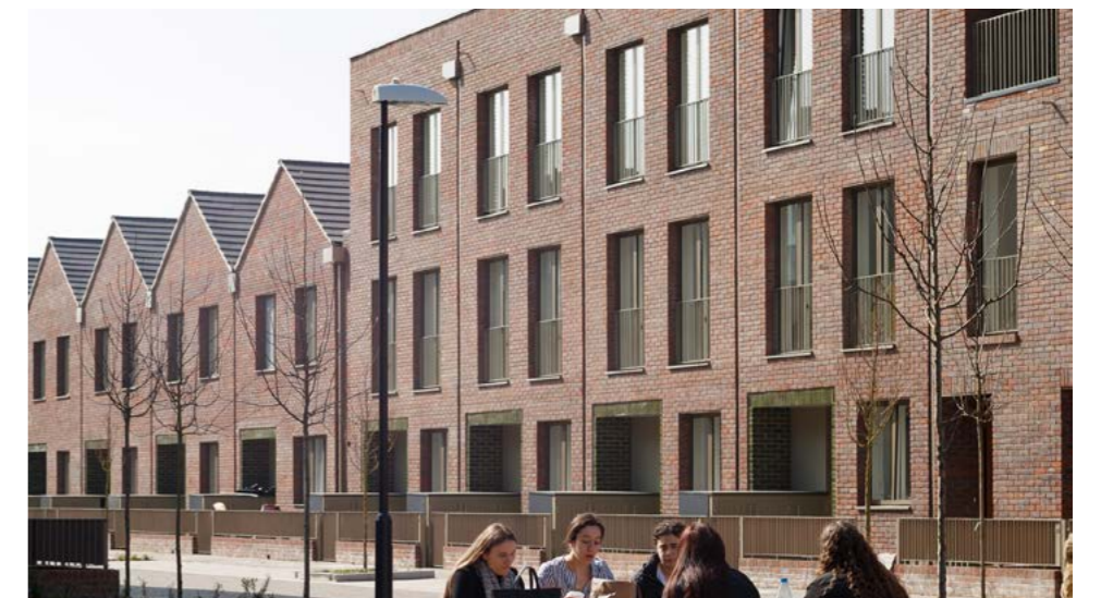
Variety of housing typologies with space for community gathering along the park, Dujardin Mews, Enfield
