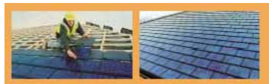
Above: Installation of PV tiles on a roof
